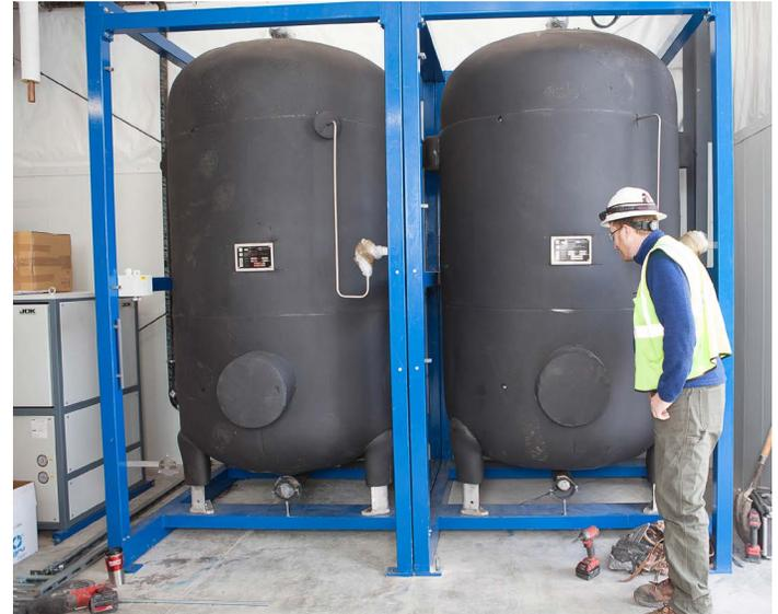
John Keefner, Underground Operations Engineer for Sanford Lab inspects activated charcoal columns, which are used to remove radon from the air.
