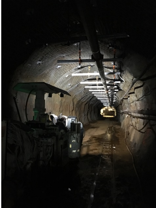
Left: Unistrut rack system
