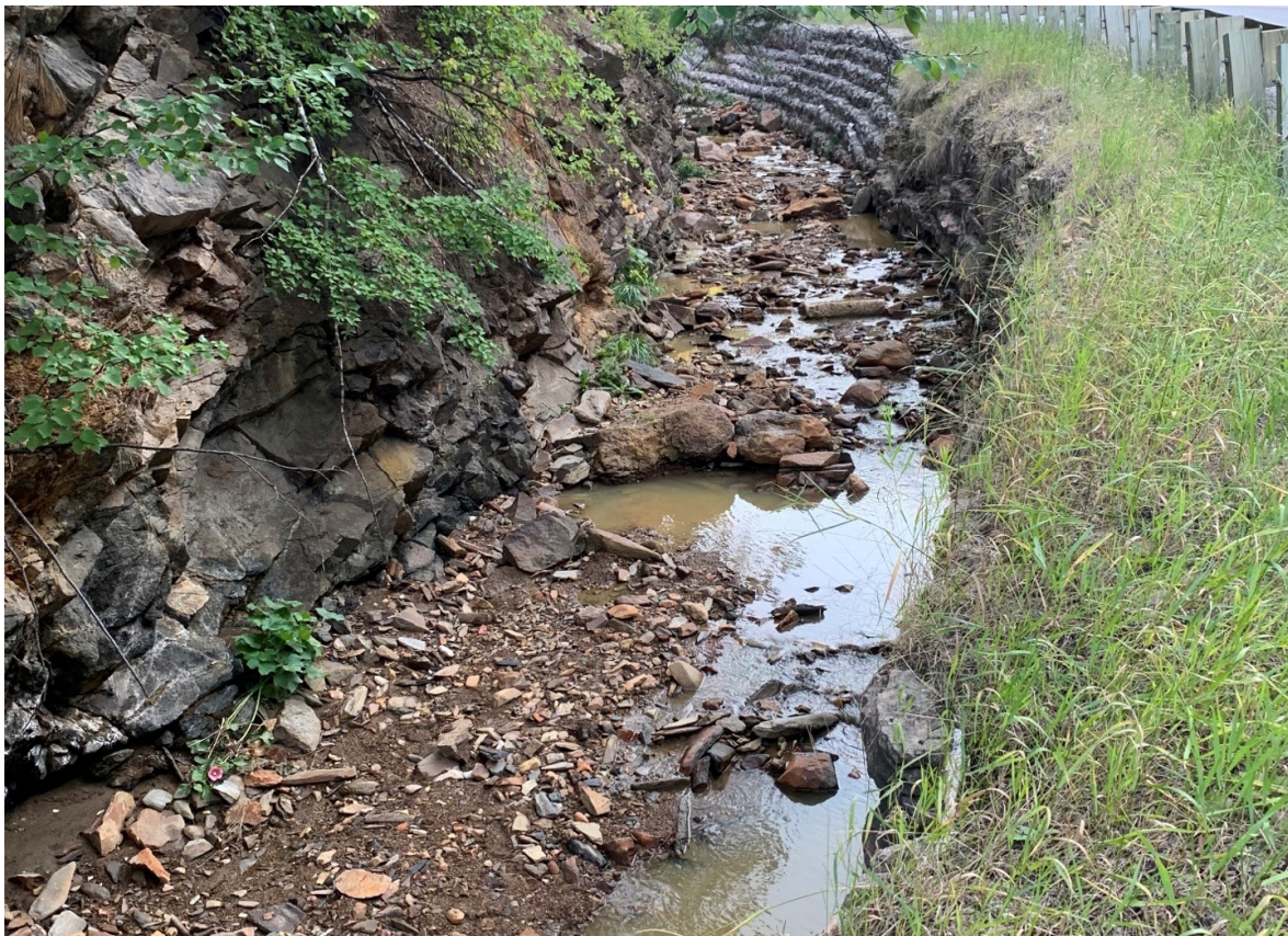
Figure 4-1: Site GR-A as viewed from the shoulder of State Highway 85, August 2021.
