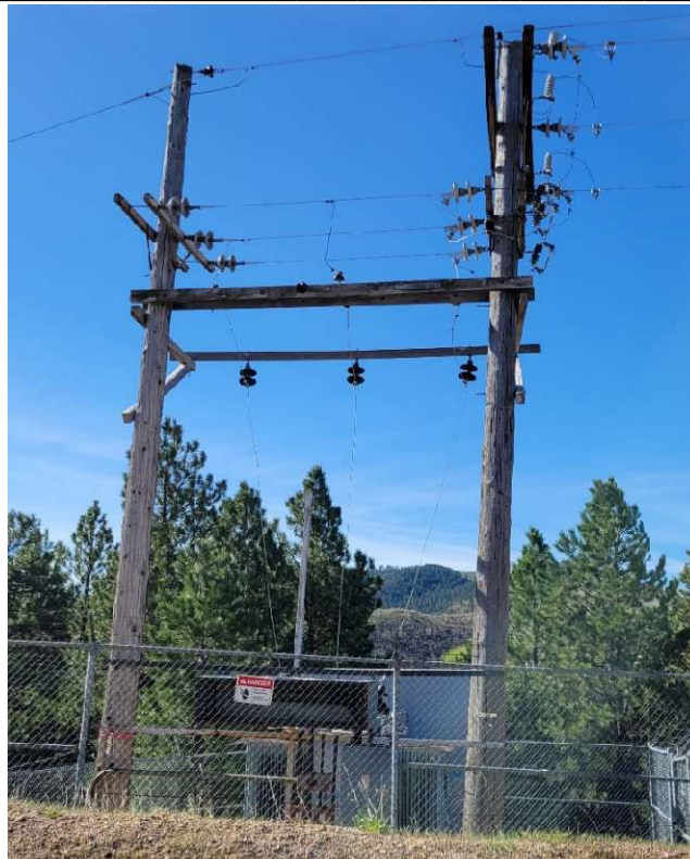
Figure 2. Picture of second structure that was visited (pole #84).
