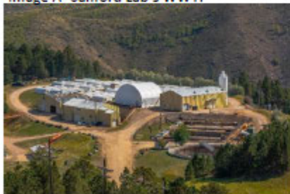
Image A- Sanford Lab’s WWTP
