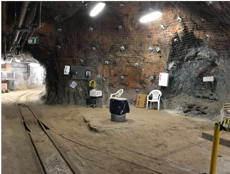
Figure 1. Future modular restroom location near #6 Winze
