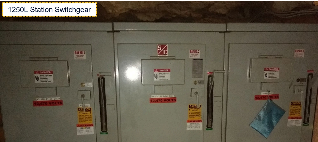
1250L Station 12KV Transformer Cage Fuse Disconnect
