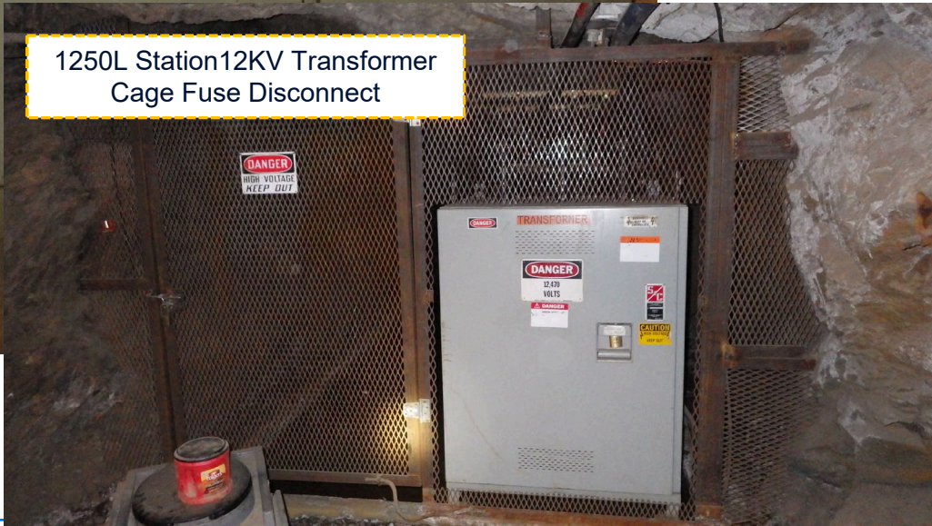
1250L Station 12KV Transformer Cage Fuse Disconnect
