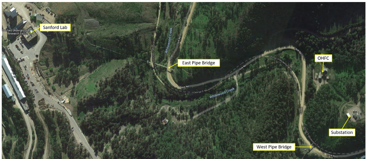
Figure 3.0 – OHFC Pipe Bridge Height Restrictions
