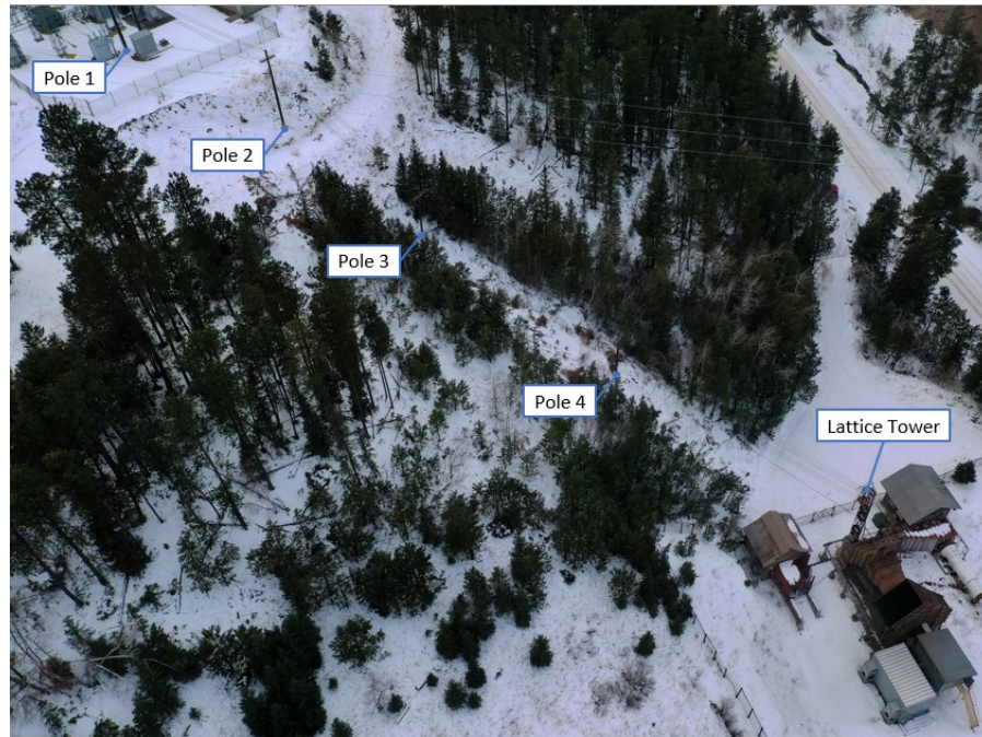
Figure 5.2 – Existing Overhead Line Feeding the OHFC
