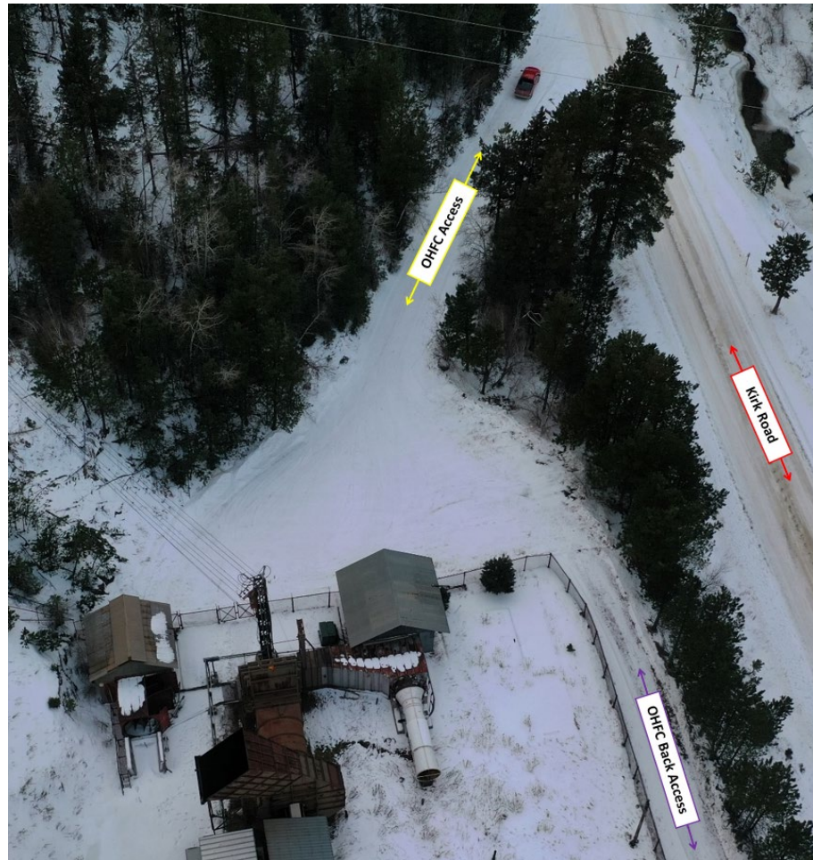
Figure 3.1 – OHFC Access Roads
