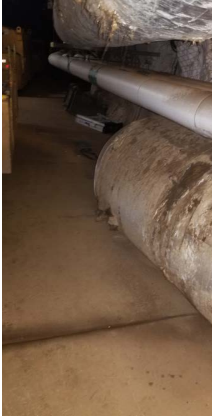
Figure 2. View of Duct Looking Down Drift
