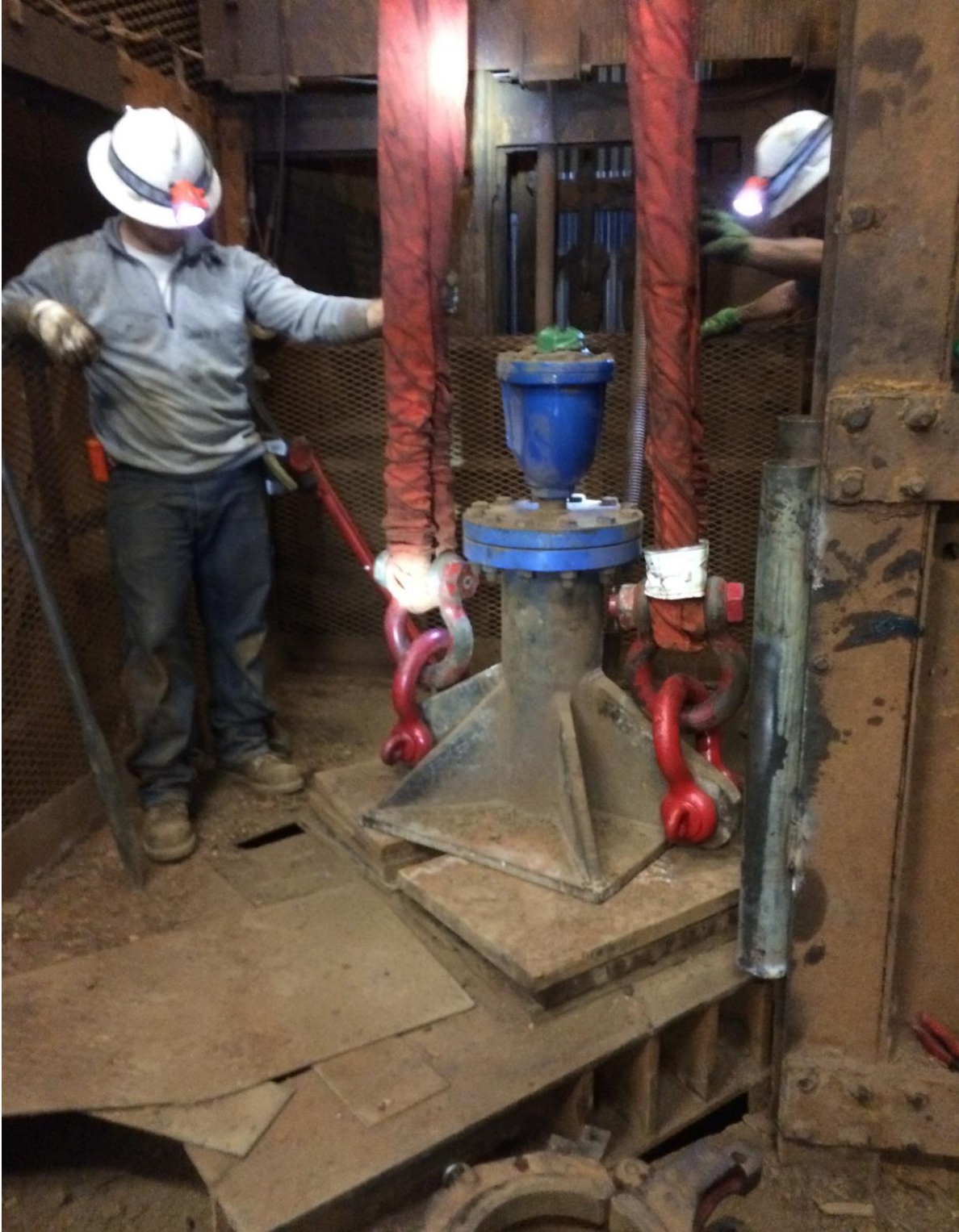
#5. WELL-HEAD BEING PLACED ON 4850L
