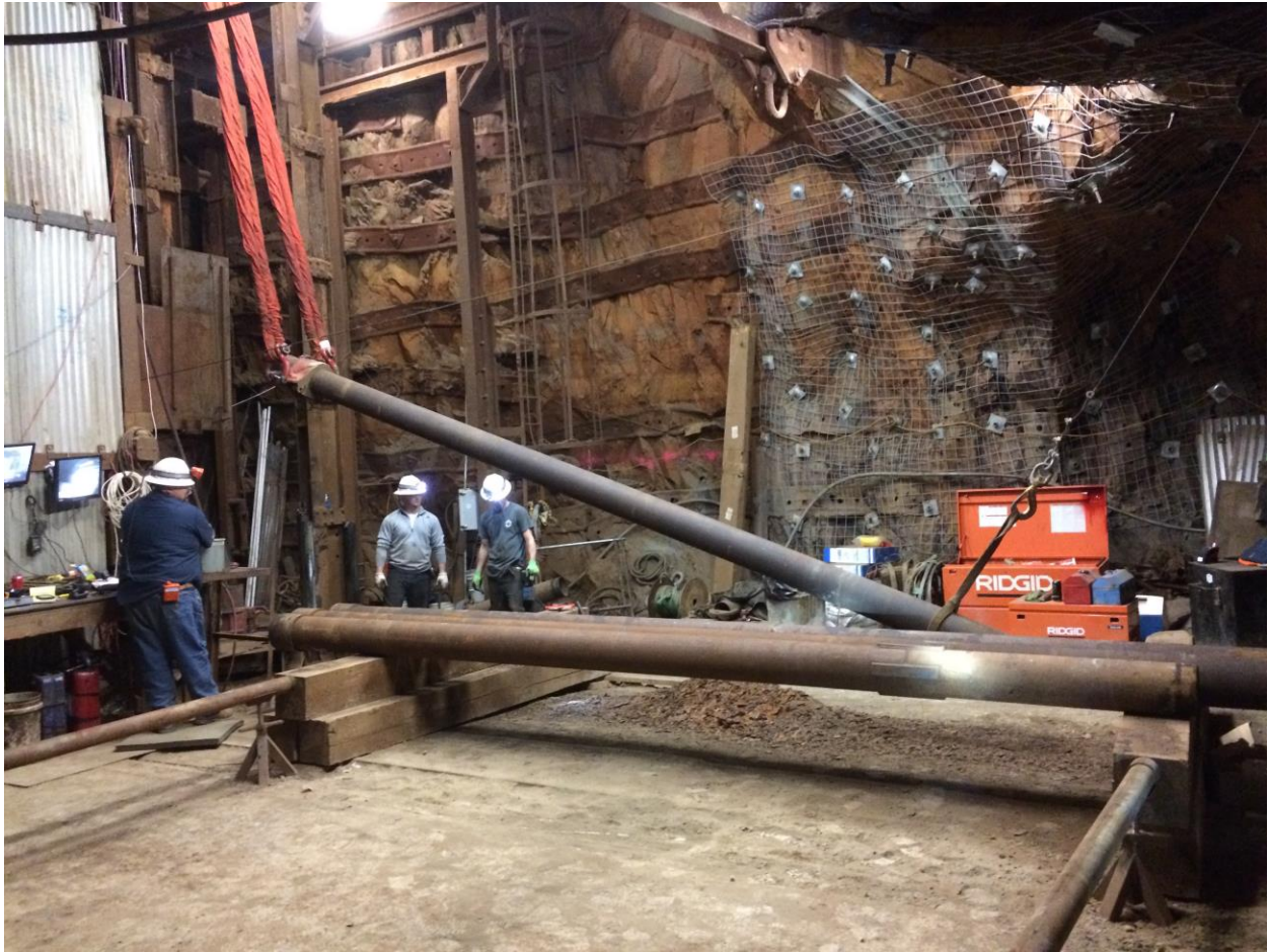
#6. USING THE WINCH, ELEVATORS, AND SYNTHETIC SLINGS TO INSTALL PIPE STRING
