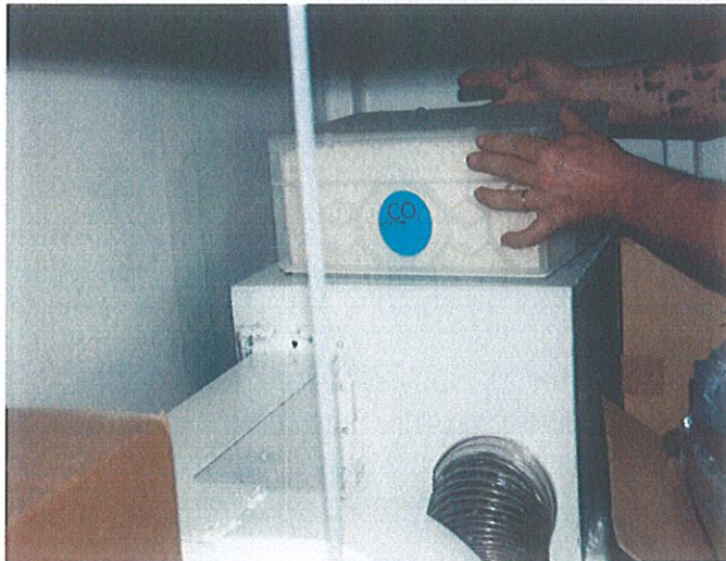
Installing CO2 Filter
