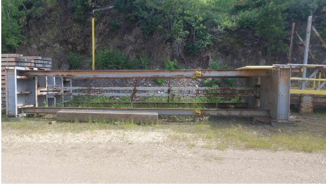
Photo #4: Upper Section of North Work Deck – Side View.
