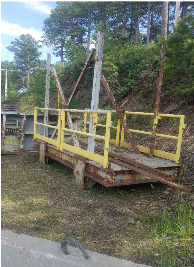
Photo #5: Lower Section of North Work Deck.
