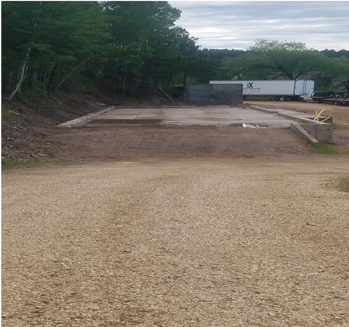
Photo #1: Rope House concrete pad – to be used as the on-site sandblasting/painting area.
