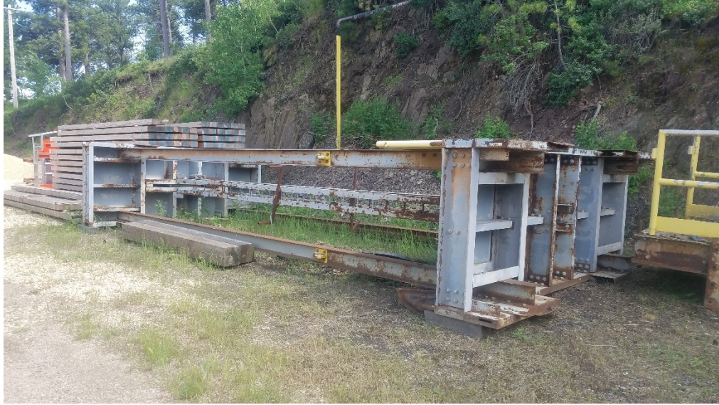
Photo #2: Upper section of North Work Deck – View from lower end.
