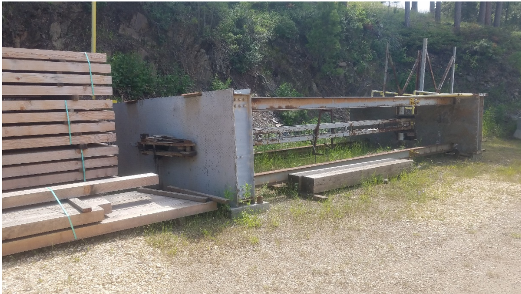
Photo #3: Upper section of North Work Deck – View from upper end.
