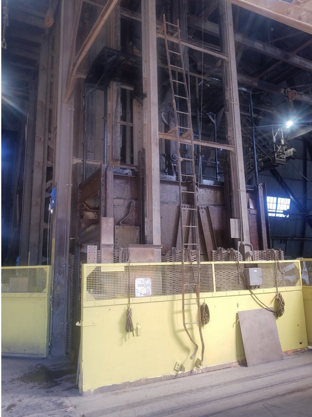
Photo #4: Yates South Cage side view. Conveyance is in the background, the Yellow perimeter guard is not part of the SOW.
