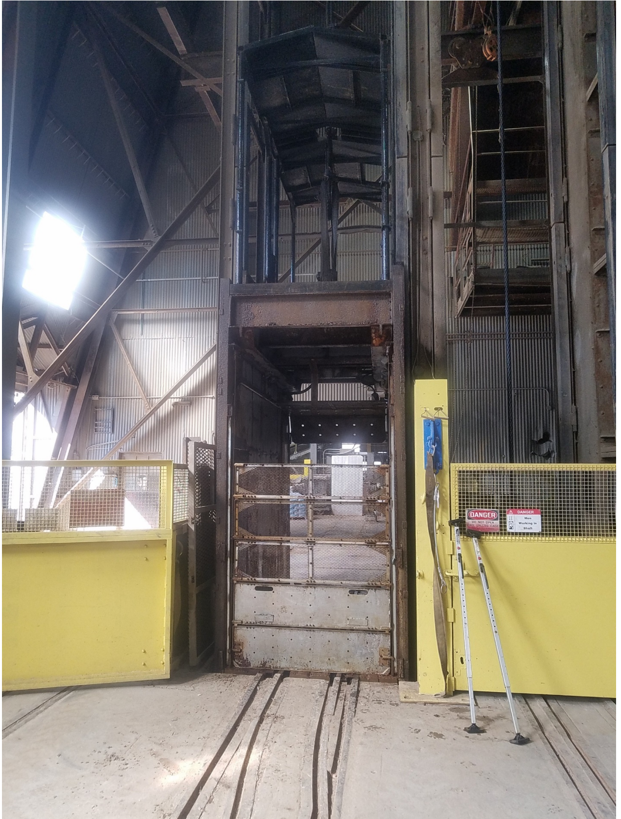
Photo #3: Yates South Cage with one of the roll-up doors closed.
