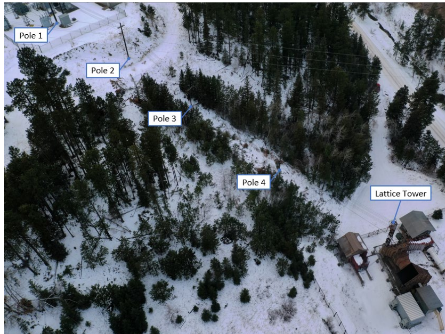
Figure 5.2 – Existing Overhead Line Feeding the OHFC
