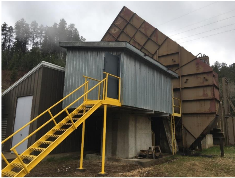
Figure 3 Drive and Motor Building Locations
