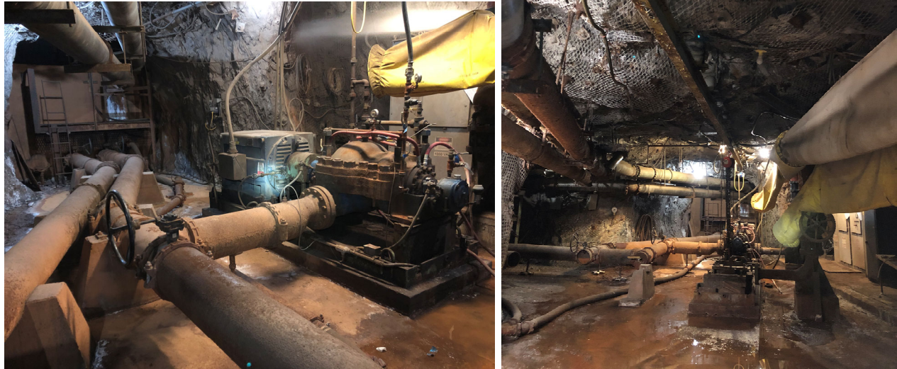
Figure 1. Existing pump and motor (left) and 3650 pump room (right)
