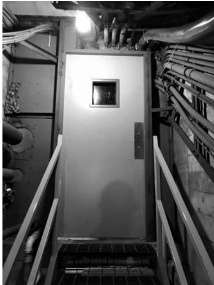
Y025 TUNNEL SIDE
