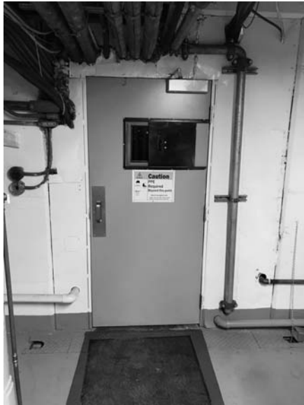
Y025 HOIST ROOM SIDE
