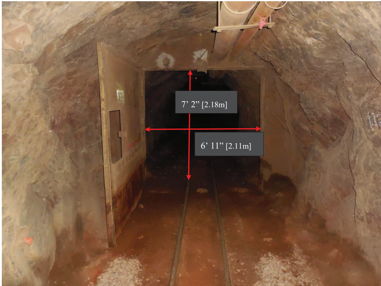
Figure 21: East Drift Access Door
