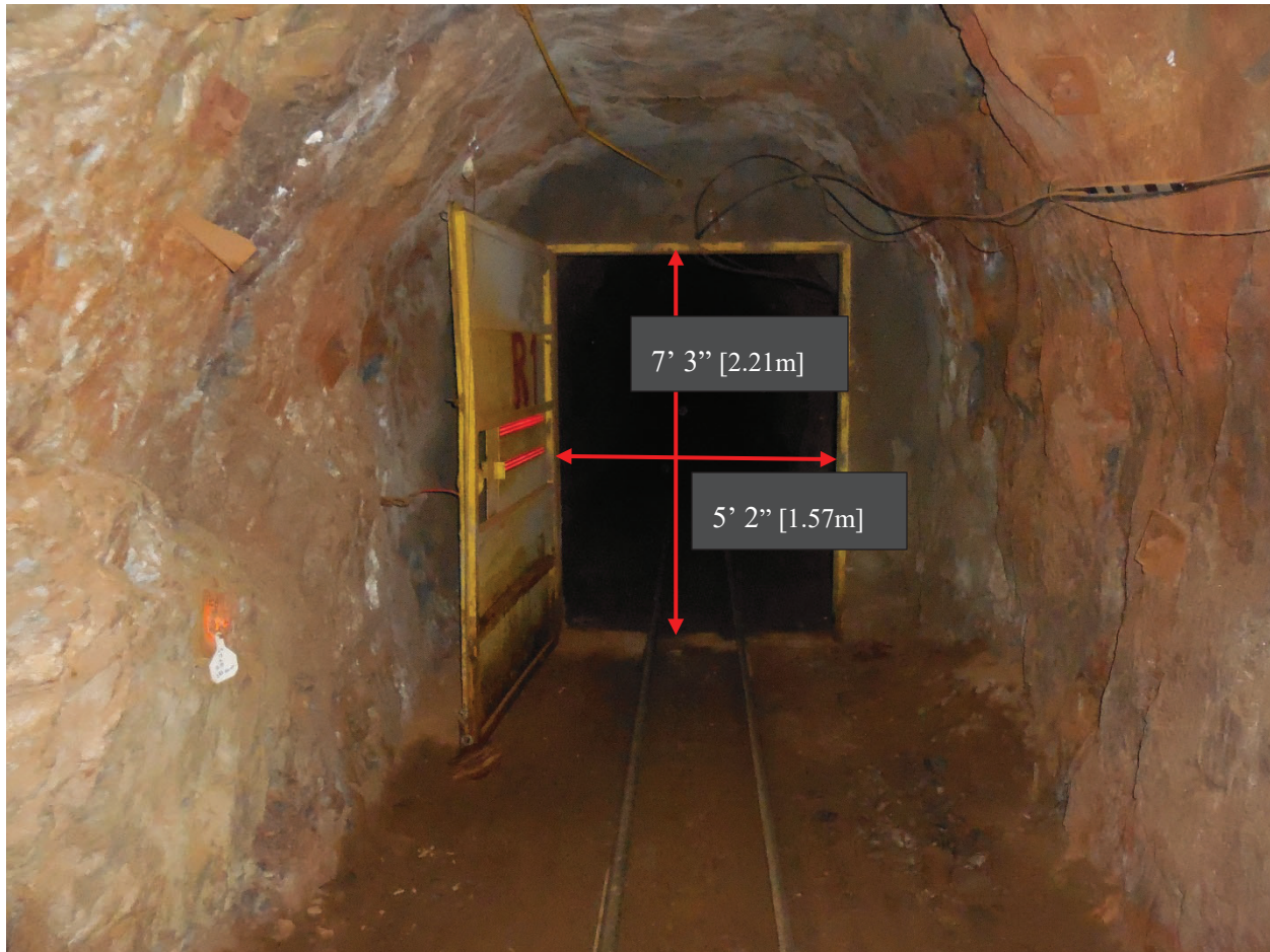
Figure 22: South Drift Access Door
