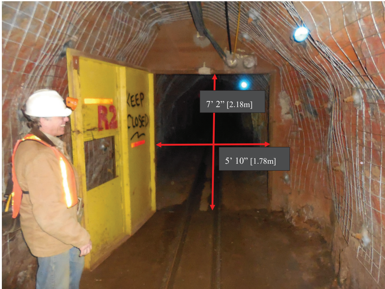
Figure 23: Ross Shaft Access Door
