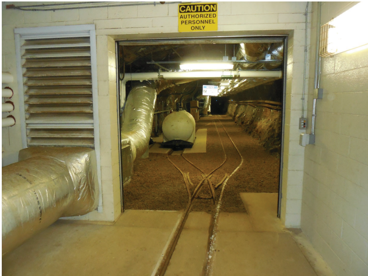
Figure 20: West Drift Overhead Access Door
