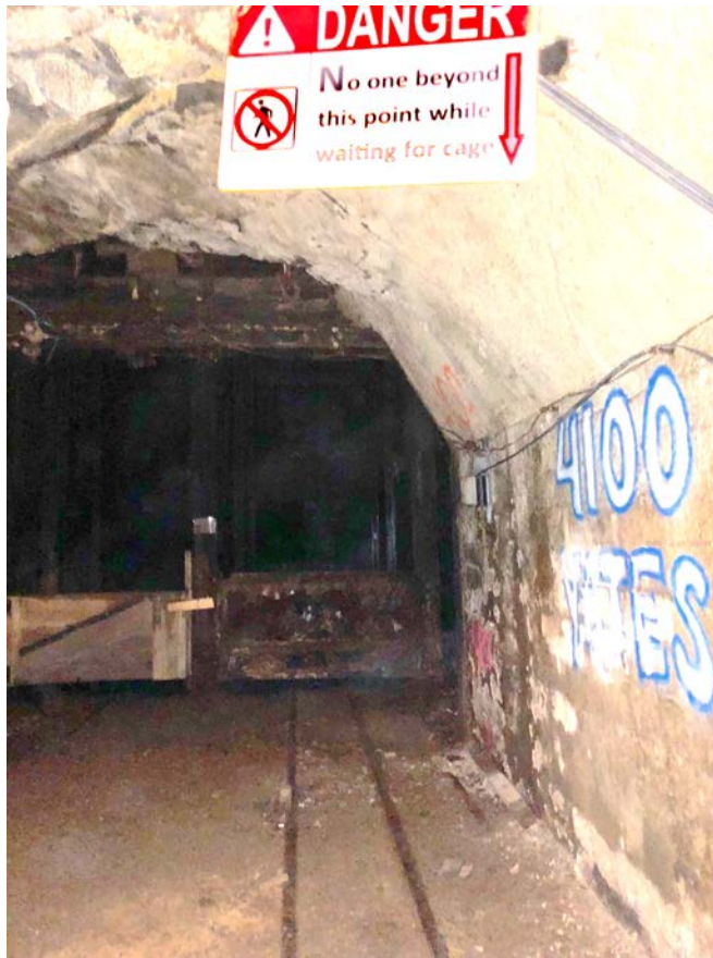
1) Looking Towards the Shaft
