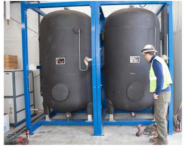
John Keefner, Underground Operations Engineer for Sanford Lab inspects activated charcoal columns, which are used to remove radon from the air.
